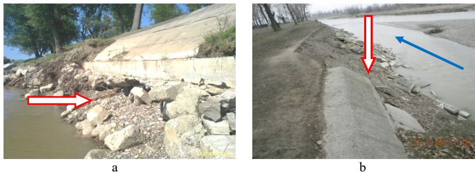
Fig. 9. Images of the protection works on the Moldova River: a - degraded left bank defence (2012); b - total left destroyed defence (year 2012) (Luca M., 2012).
